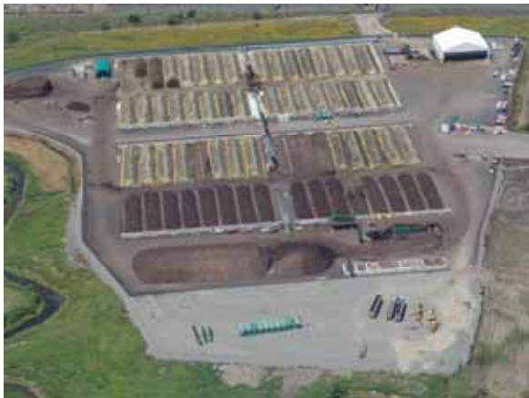
200,000 tpa plant in Seattle
